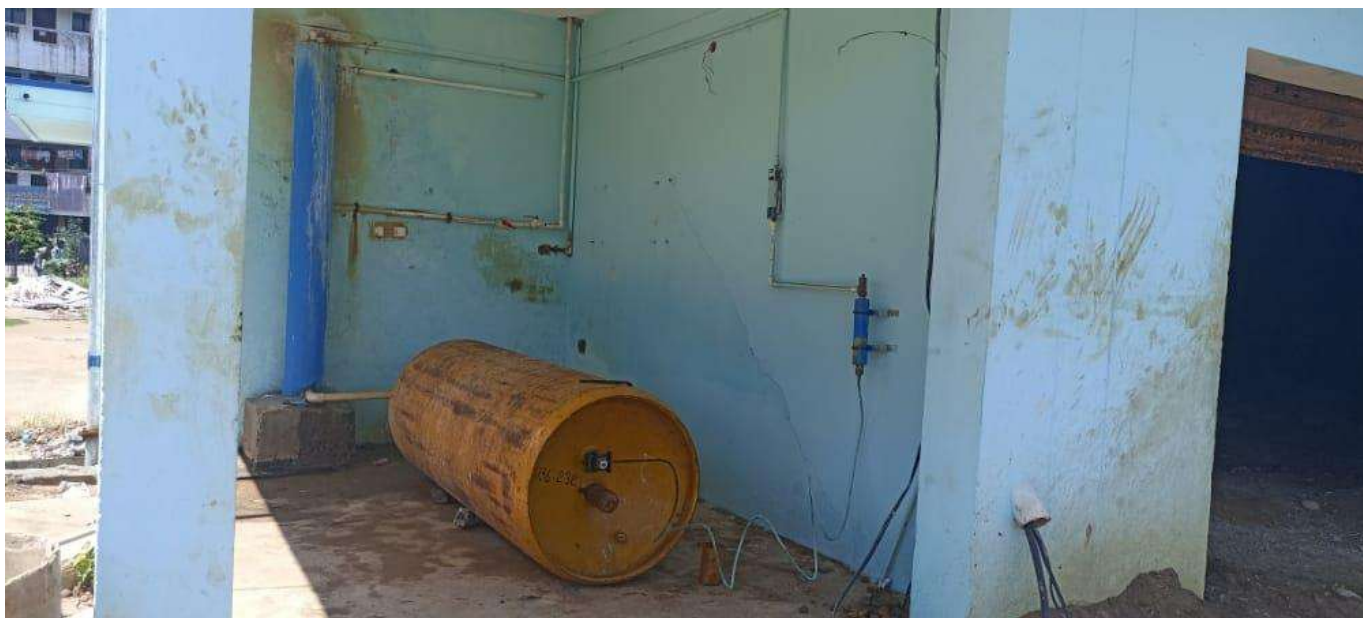
Fig: 7 Chlorine cylinder for chlorination of water (chlorine pumped through the pipes to the filtered water for disinfection)
