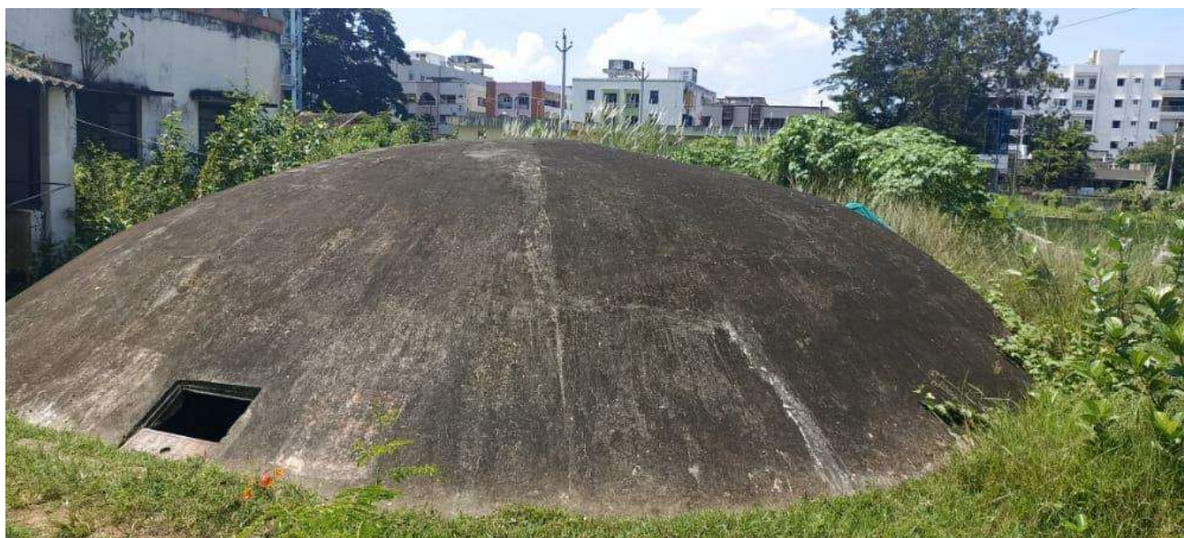
Fig: 8 Chlorinated water stored in the tanks for checking the ppm of Chlorine before supply
